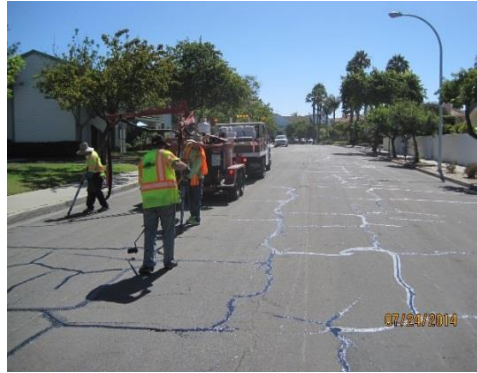
Crack seal
