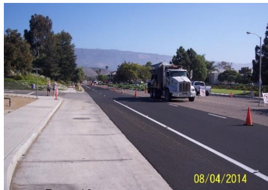
Cape Seal (Chip Seal Placement)
