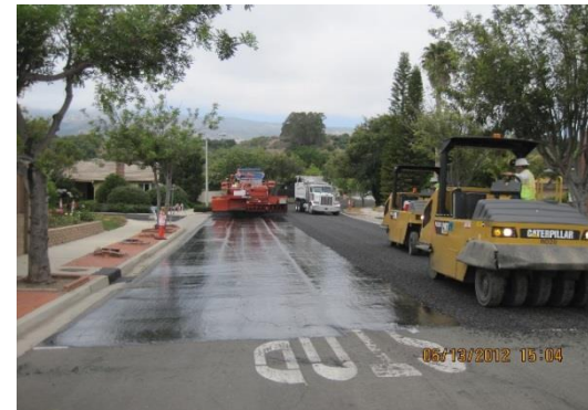
Cape Seal (Chip Seal Placement)
