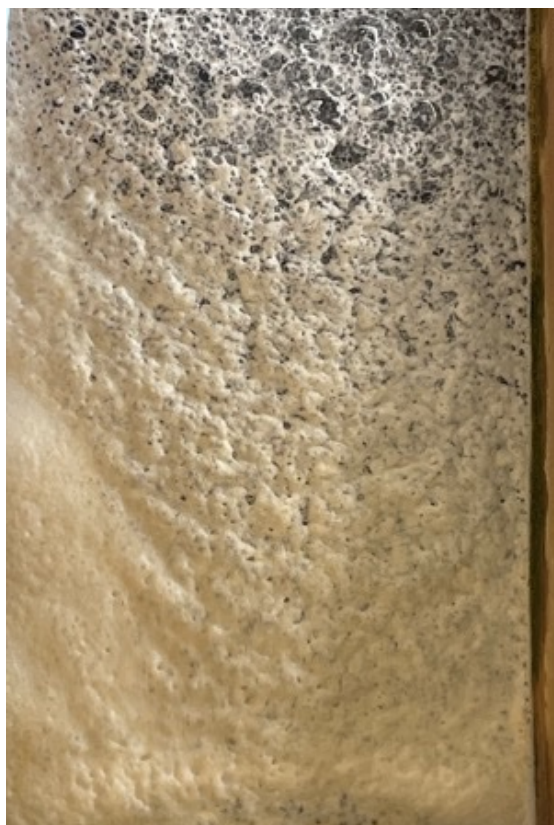
Figures 7-9. Scum collecting at the top of collection tanks within 24 hours of IOC commencing.
