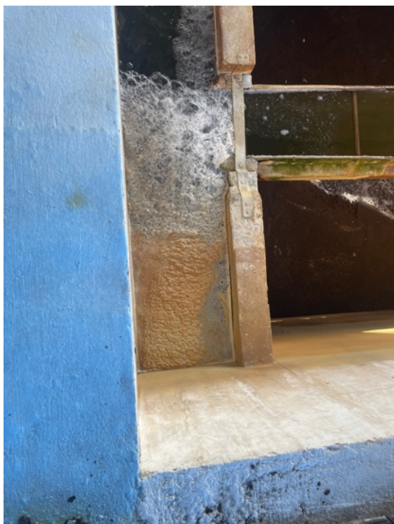
Figures 7-9. Scum collecting at the top of collection tanks within 24 hours of IOC commencing.
