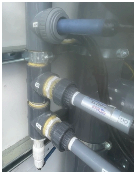
Figure 12. In-line sensors provide real-time ORP, pH, DO, and TDS measurements.
